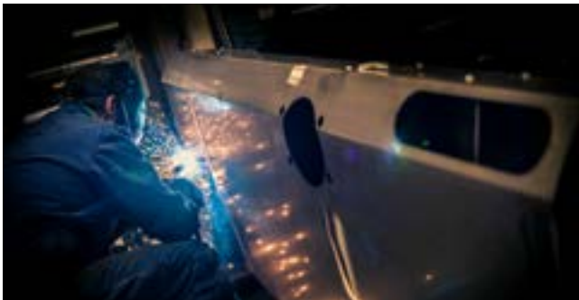
Welding of frame
