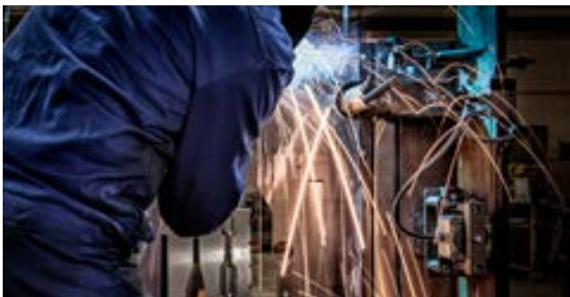
Welding of frame
